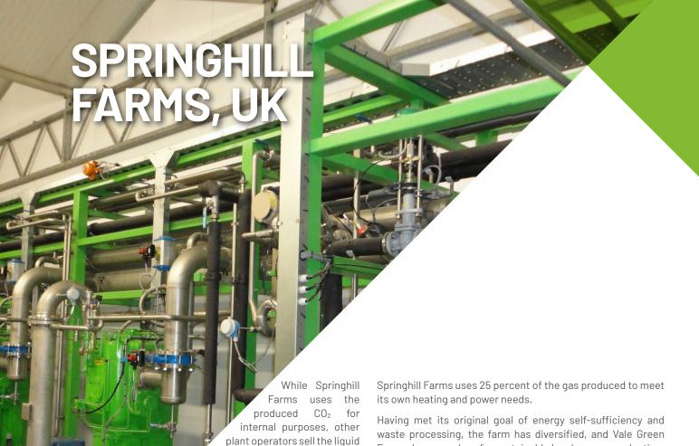
Since August 2013, Springhill Farms has delivered biomethane to the Wales and West Utilities gas grid. At full capacity, the system produces 225 Nm<sup>3</sup>/h of biomethane 24/7, which is enough to supply 1,000 households with their annual natural gas consumption.
